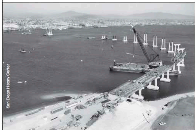
Construction of the Coronado Bridge, circa 1969
